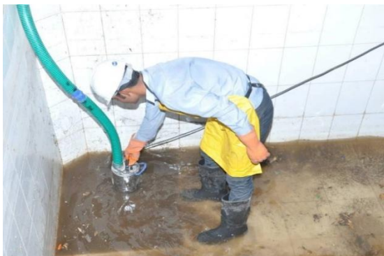
Fig. WTC_M.3.20 Draining Wastewater
