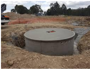
Concrete Underground Water Tanks
