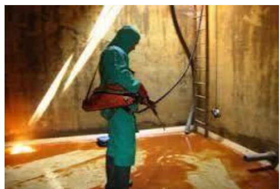
Fig. WTC_M.3.21 Pressure Cleaning
