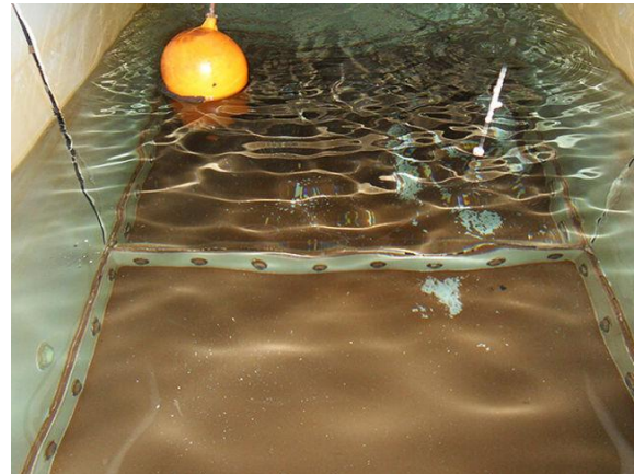
Fig. WTC_M.3.4 Sign of Contamination
