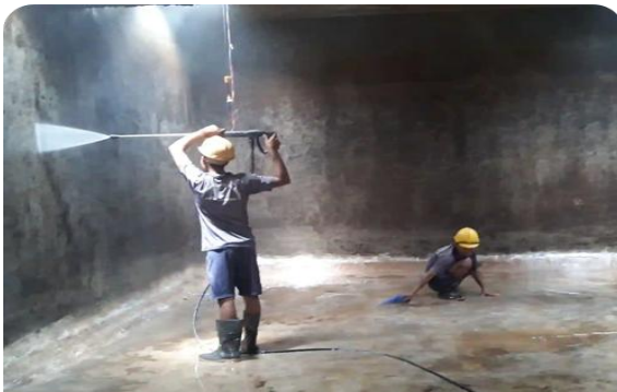
Fig. WTC_M.3.18 Pressure Washing
